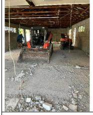
be termite proofed, and a new slab will be pinned - this makes the building compliant to today's standard.
